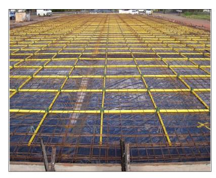
The JFS grid is currently available in two sizes. The smaller version is for slabs up to 4 inches thick, the larger version is for slabs up to 6 inches thick.
